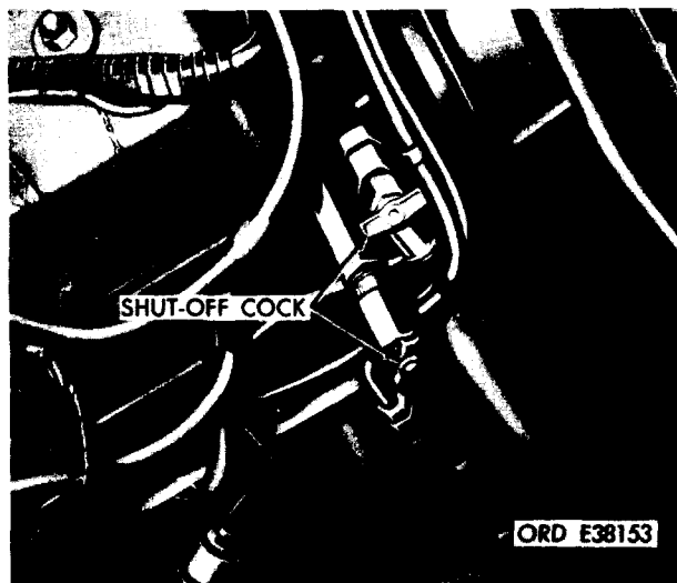
Figure 4-19. Heater shutoff cocks.
